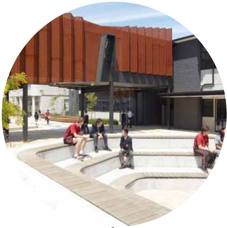
CONCRETE AMPHITHEATRE STYLE SEATING
